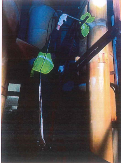
蚀刻工序废气处理后排放口 DA003
